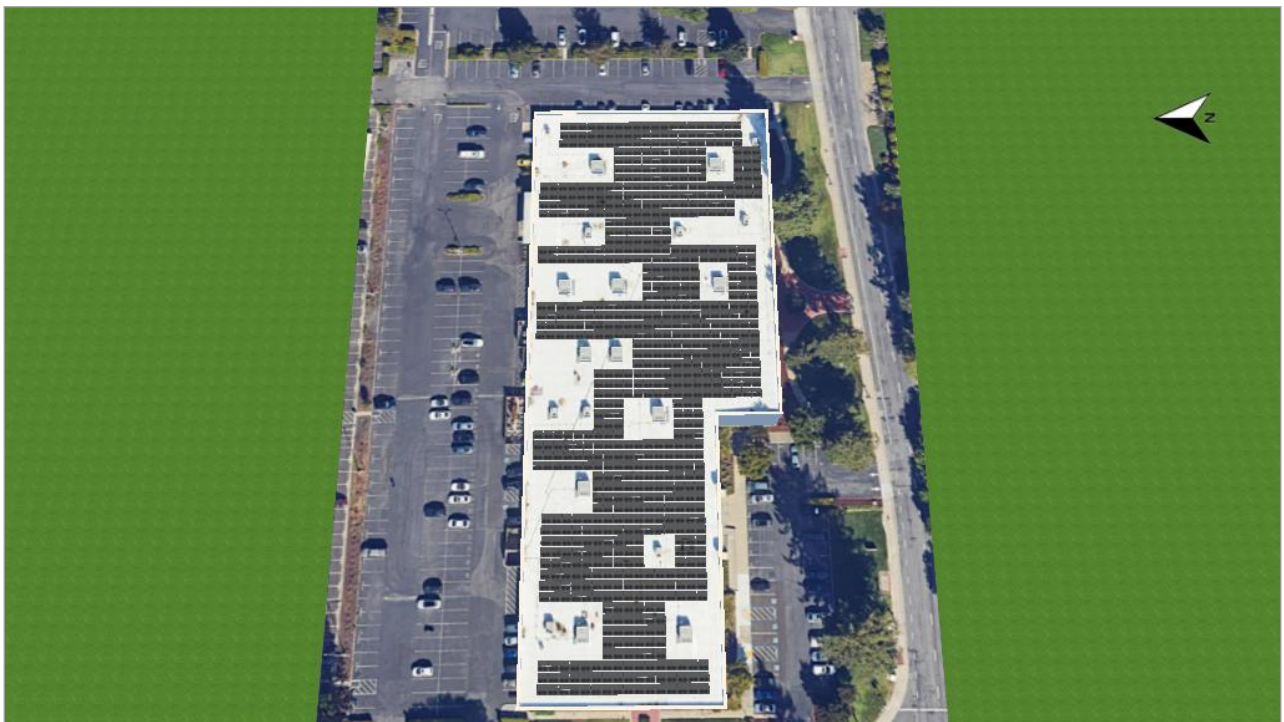
Figure: 1. Module Area - Arbitrary Building 01-Module Area West
